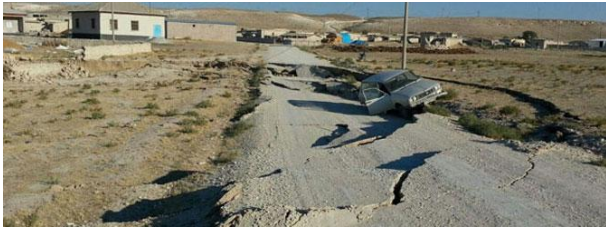
Figure 2. The earth surface fissure due to land subsidence
