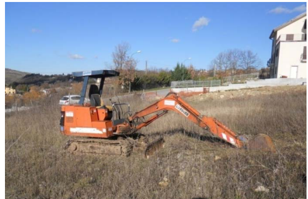
Figure 6. Mini Excavator located on 19 February and 08 April 2014
