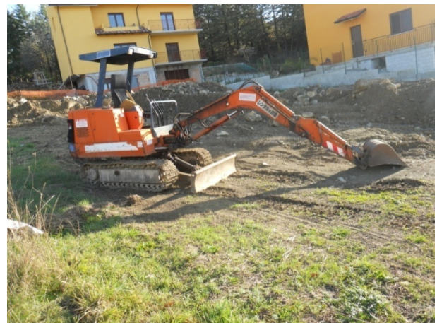
Figure 7. Mini Excavator situated on 21 and 24 November 2014
