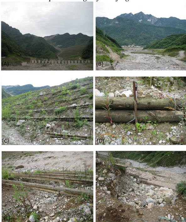
Figure. 3 Field investigation pictures of the landslide.
